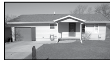
908 Walnut Street 4 Bedrooms, Large Backyard $115,000
